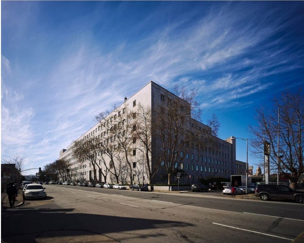
San Francisco Hall of Justice 2017 by Dllu is licensed under CC BY-SA 4.0 .
