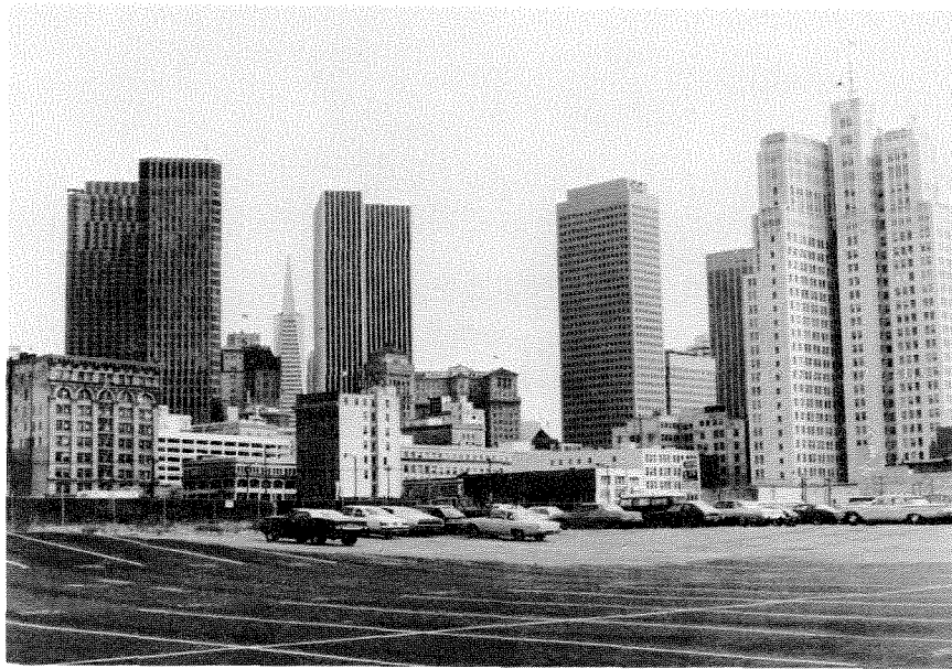
PHOTO 5 Looking Northeast from CB-2, with the Mercantile Building in the left foreground
