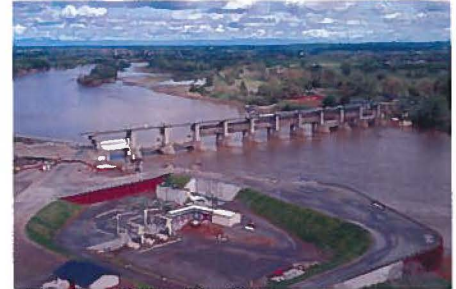
Red Bluff Diversion Dam
