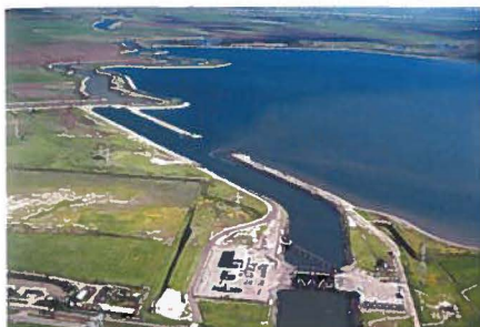
Clifton Court Forebay
