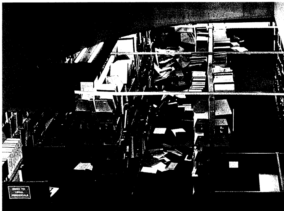
Unbolted shelves moved and hundreds of books fell to the Law Library floor during the 1989 Loma Prieta earthquake.
